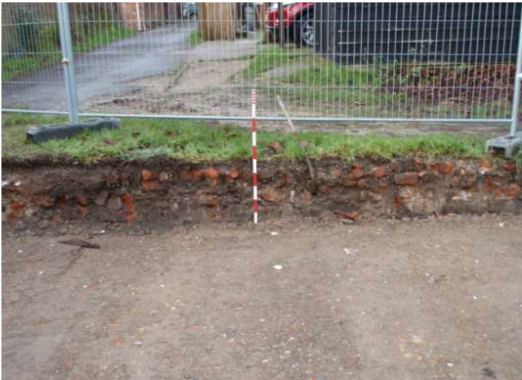
Plate 5. Reduction of Area 1 (Phase 2) completed and Type 2 rolled in ready for building slabs (looking west)
